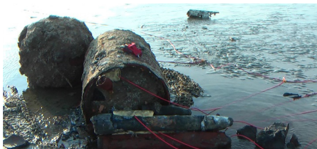
Various munitions that were cleared during a shipping line extension in the German North Sea are prepared for detonation at low tide (Photo: SeaTerra).
